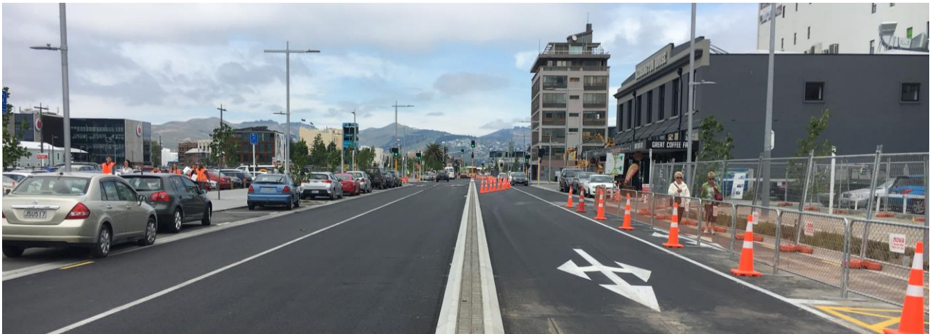
Part of the recently completed road surface on Manchester Street.
